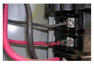
One of the worst things found in a panel is **overheated wiring**, like this panel above. This is an indication of either too many circuits connected to this breaker, possibly a defective breaker, or a wiring problem causing arcing. This is a big safety issue that will need investigated immediately, to prevent the risk of a fire developing.
