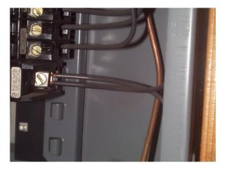
The other common item is **double-tapping of breakers**, where two wires are connected to one breaker. This can overload a circuit, and can also lead to arcing in the panel, if one of the connections is not tight.
